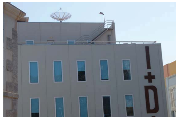
Figure 13. Final emplacement of the SRT at UPCT.
