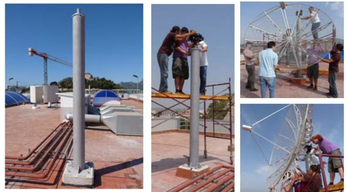
Figure 11. Emplacement of the engines and antenna at post.
