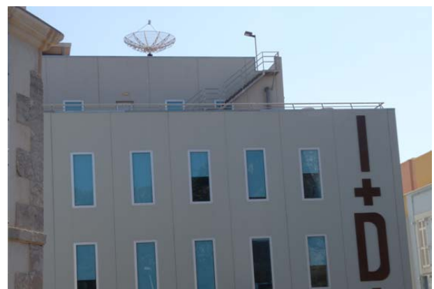
Figure 13. Final emplacement of the SRT at UPCT.
